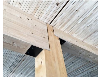
Figure 4. Structural connection detail using wood [see footnote 24].
