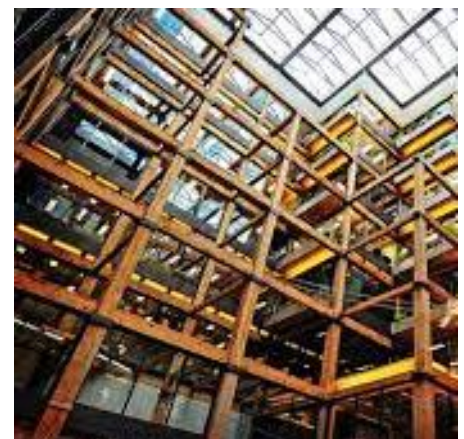
Figure 3. Construction of multi-story building using wood [see footnote 23].
